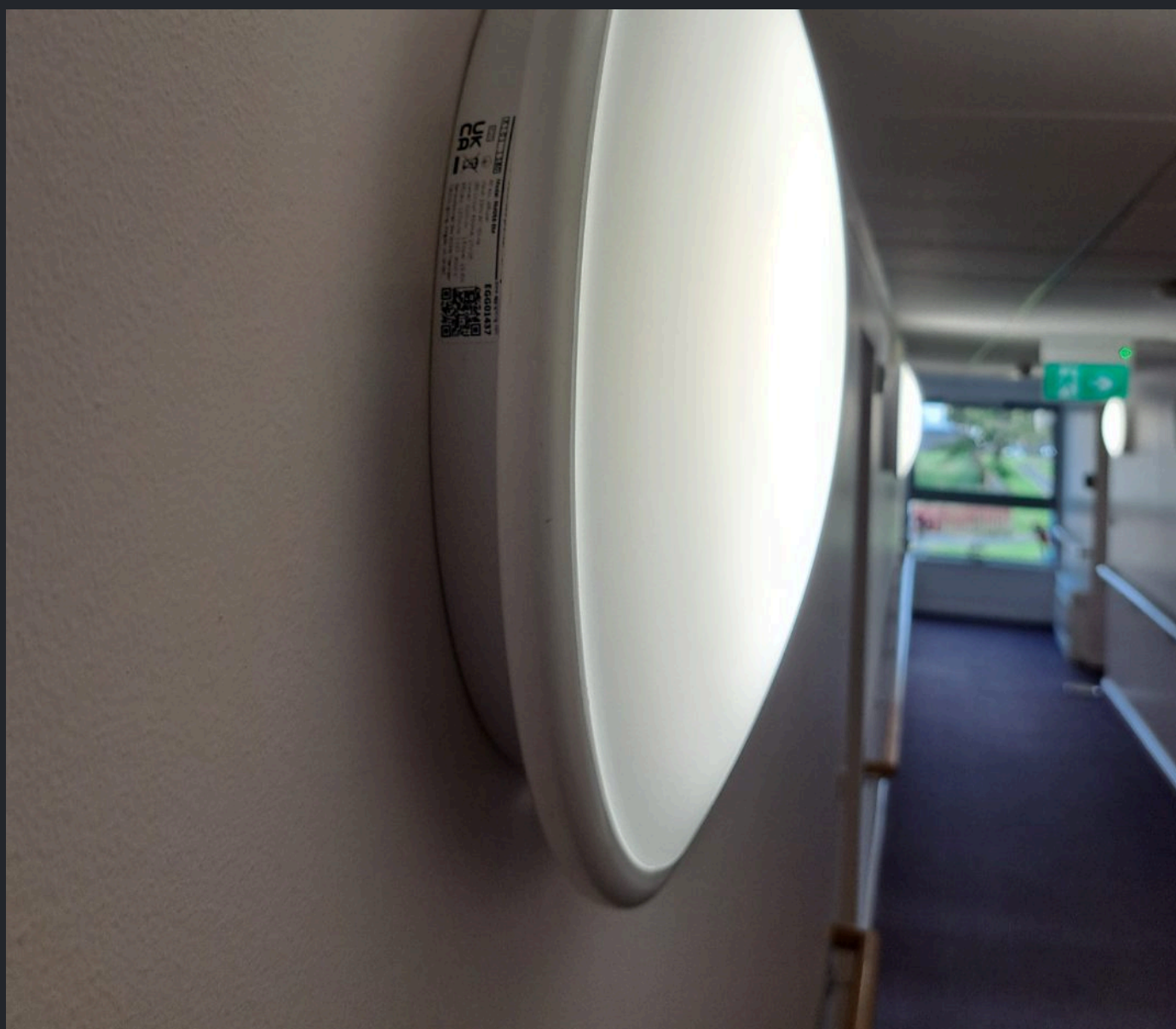
Mission Place, Motherwell — a communal corridor after installation.
